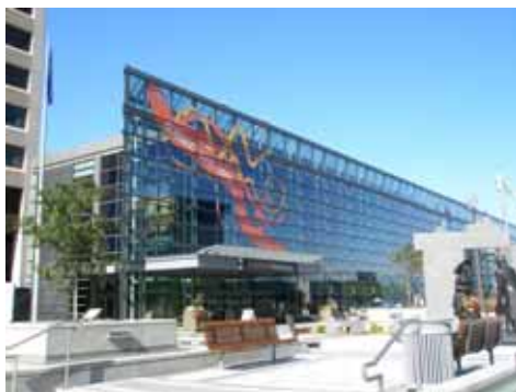
Convention Centre (写真1)
