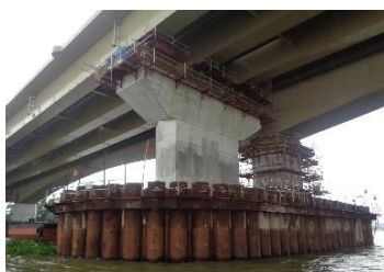
Steel Pile Sheet Pile
