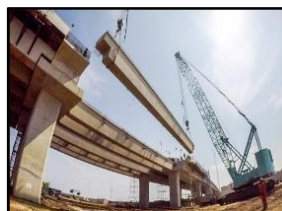
U-Girder Erection
