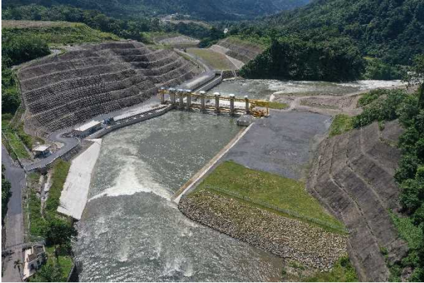
Intake Weir and Facilities
