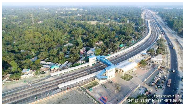
Completed Station and Platform
