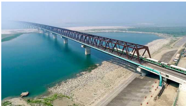
Completed Railway Bridge
