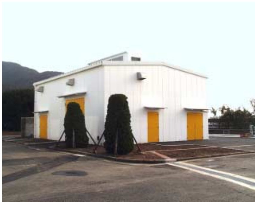
Fig. 4.2.3-2 External View of Laboratory Building
